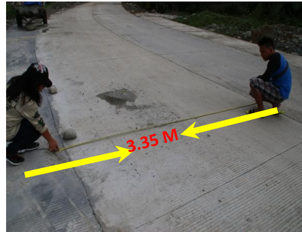
Constructed PCCP must conform with the approved POW/design
